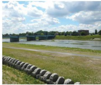
From Top River Run, Wolf Creek crossing, Existing retaining wall
